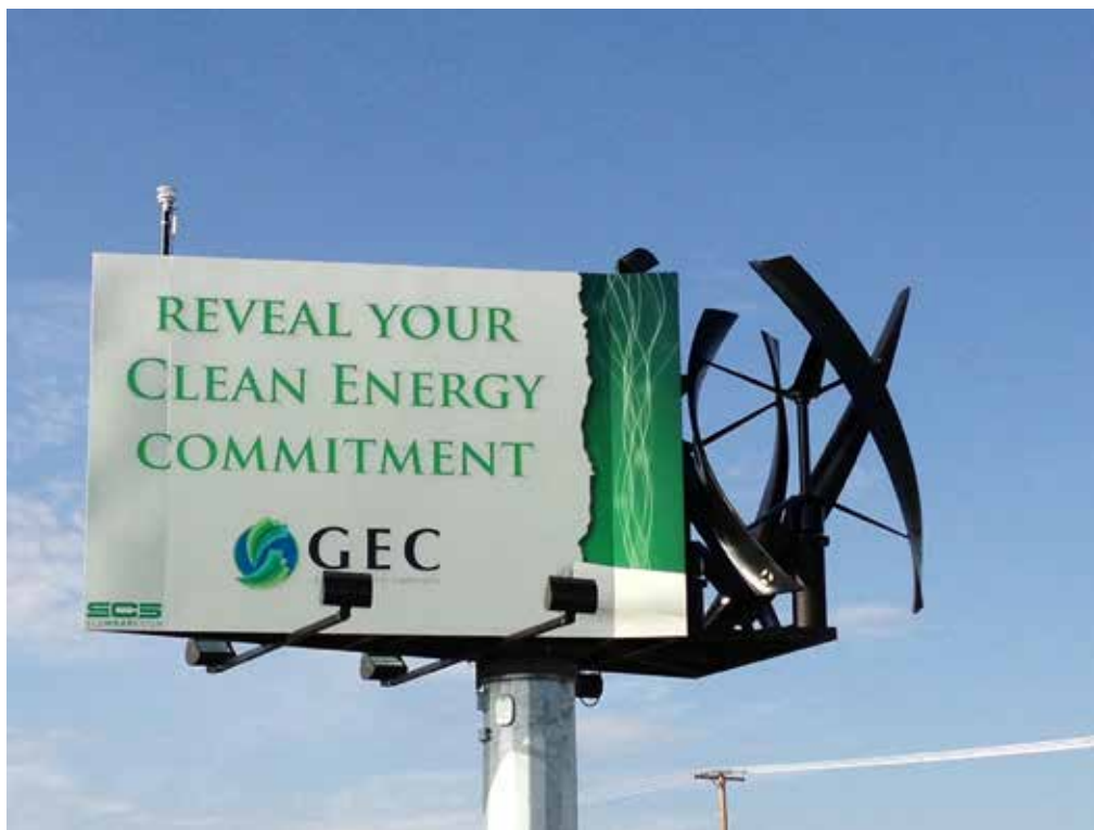
Wind energy from this Montana billboard is a distributed energy resource (DER)
