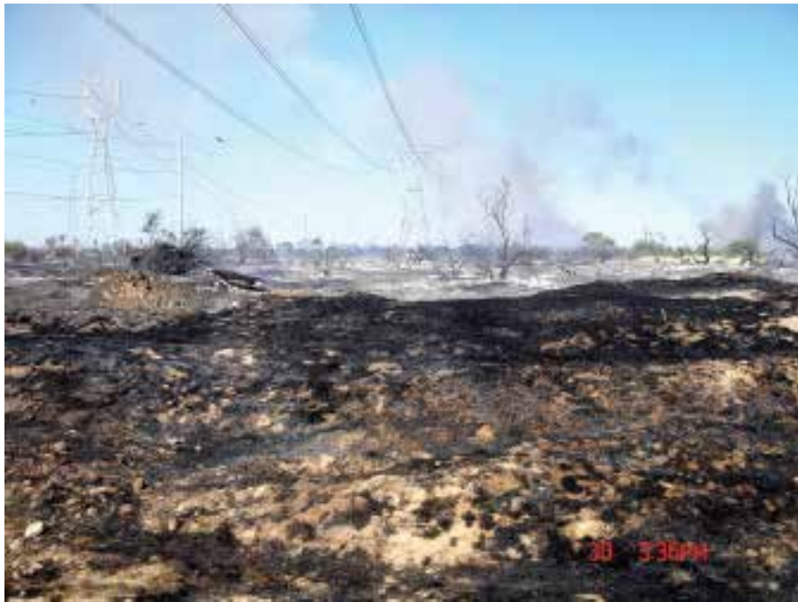
June 2005 wildfire in southwest Phoenix, Arizona area causing out-age on six circuits of 500kV, 345kV and 230kV transmission lines.
